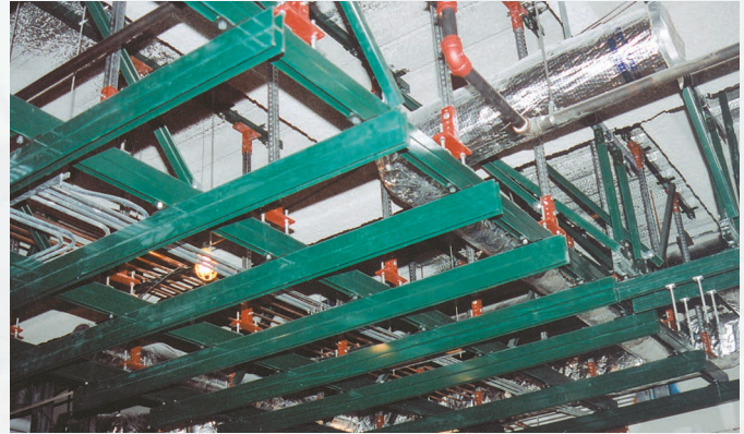
Multi-rail support system with Telespar drops.
